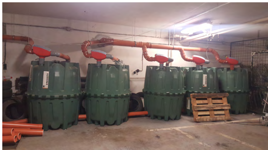
Water tanks in the basement of the City Municipality building, collecting the rainwater, which is afterwards used for flushing lavatories. Zvolen, Slovakia (Photo: Maria Bihunova)
