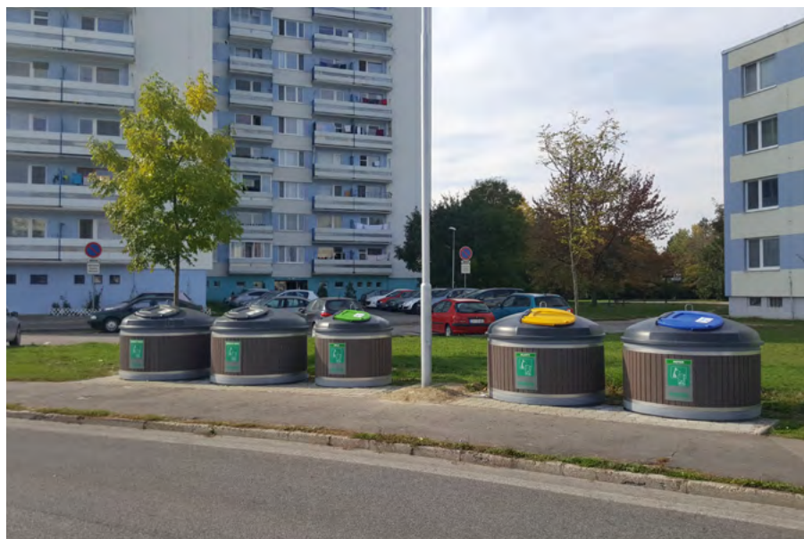
Example of the municipal waste treatment, the waste underground tanks, which can signalise when they are getting filled, Nitra, Slovakia (Photo: Maria Bihunova)
