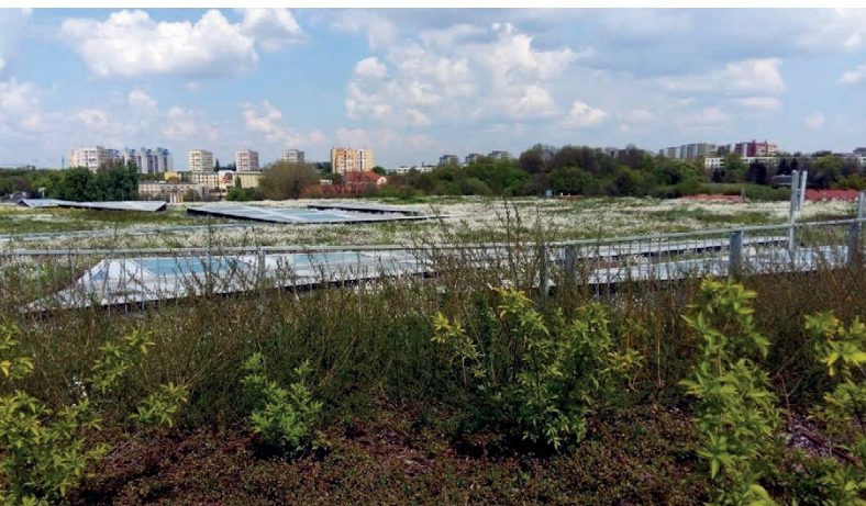
Photo 1. Extensive roof at Galeria Vivo! in Lublin, 2018 (photo M. Dudkiewicz)
