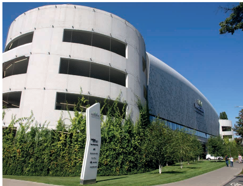
Photo 1. Creepers climbing a steel mesh stretched on the concrete facade of the building. Multi-storey car park in the Wroclavia shopping gallery at Joannitów str. in Wrocław (Author's collection)
