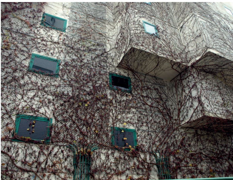
Photo 2. Concrete facade with creepers on a steel mesh. A local car park at Stanisława Herbsta Str. in Warsaw (Author's collection)
