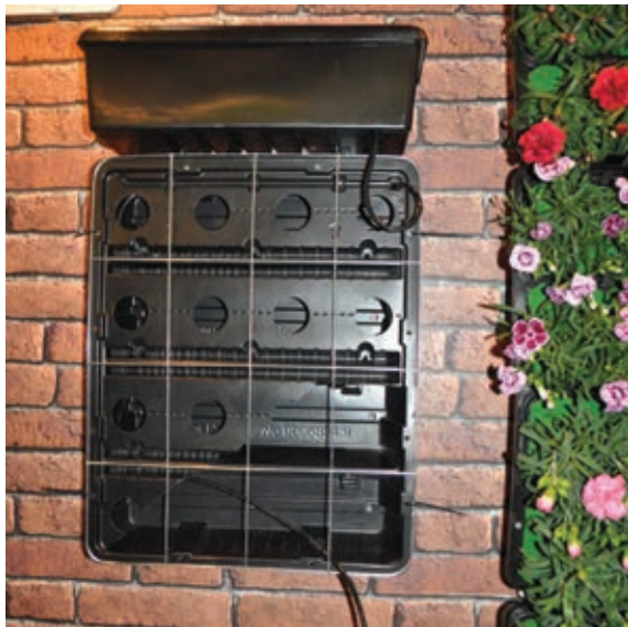
Fig. 3. Construction of panels (trays) Fig. 4. A living wall made by trays
