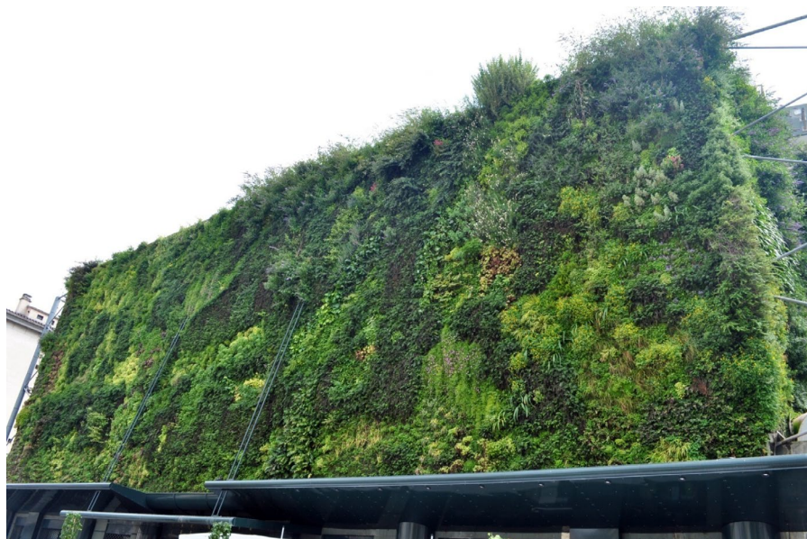
Fig. 2. Continuous living wall (photo by M. Weber-Siwirska)
